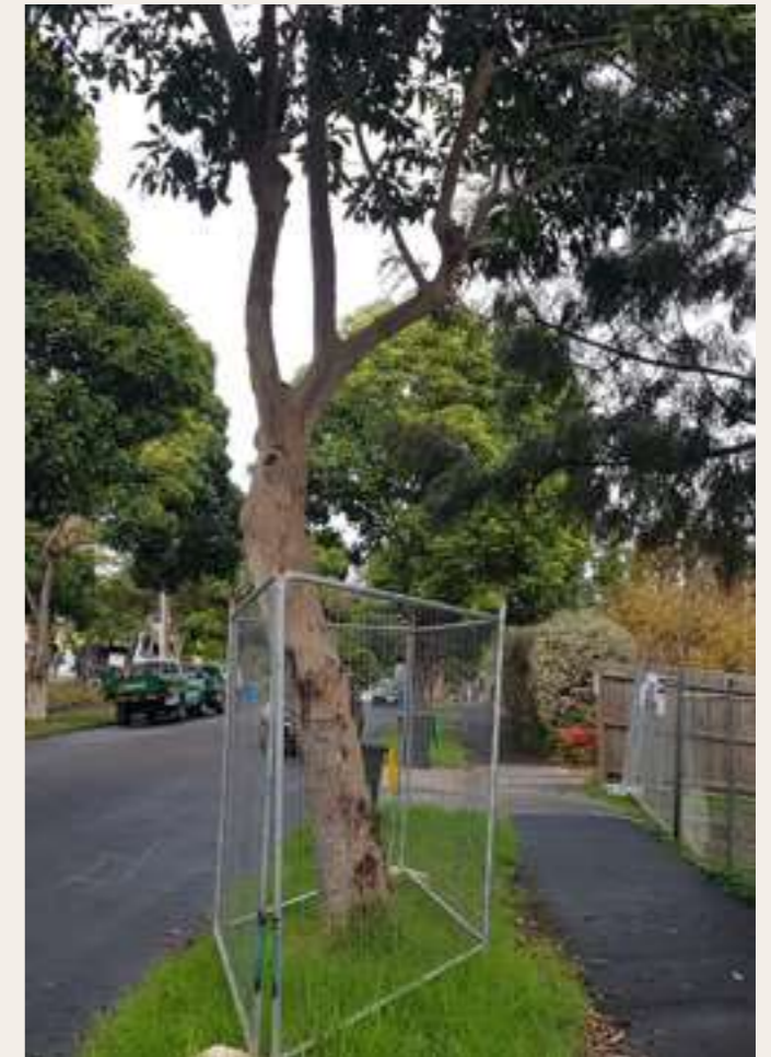
Above: Tree protected on nature strip prior to works
